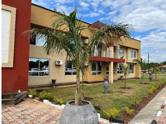
Administration building of the NCS
